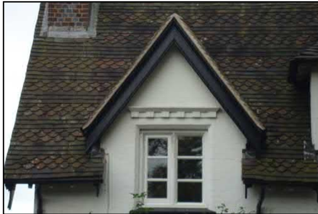
Figure 52: Decorative window headers
