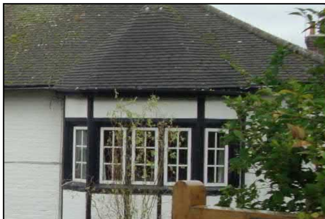
Figure 54: Windows maintain the traditional sub-division of panes
