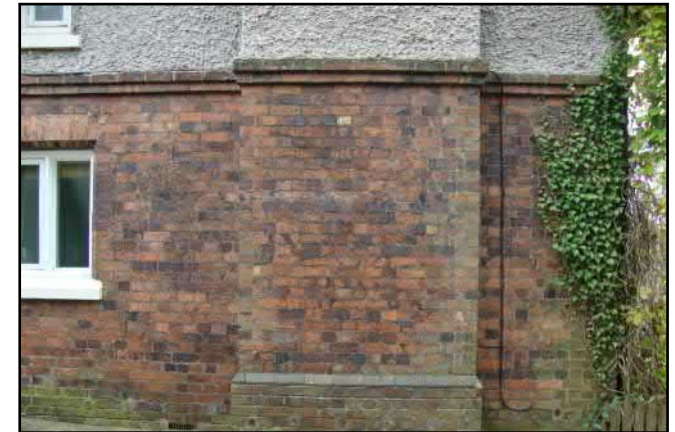
Figure 53: Fine red and blue brickwork
