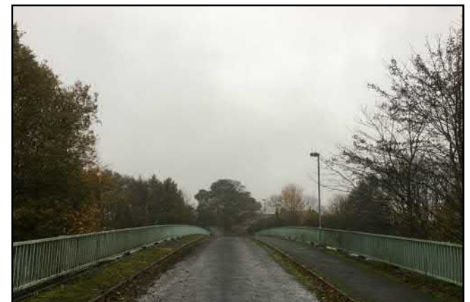
Figure 12: PRoW - Bridge over A525
