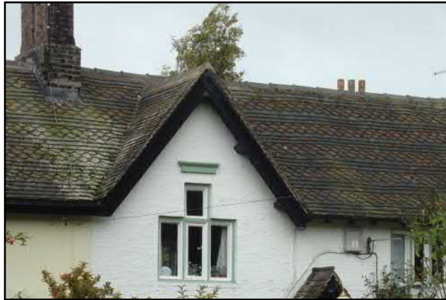
Figure 50: Patterned fish scale roof tiles
