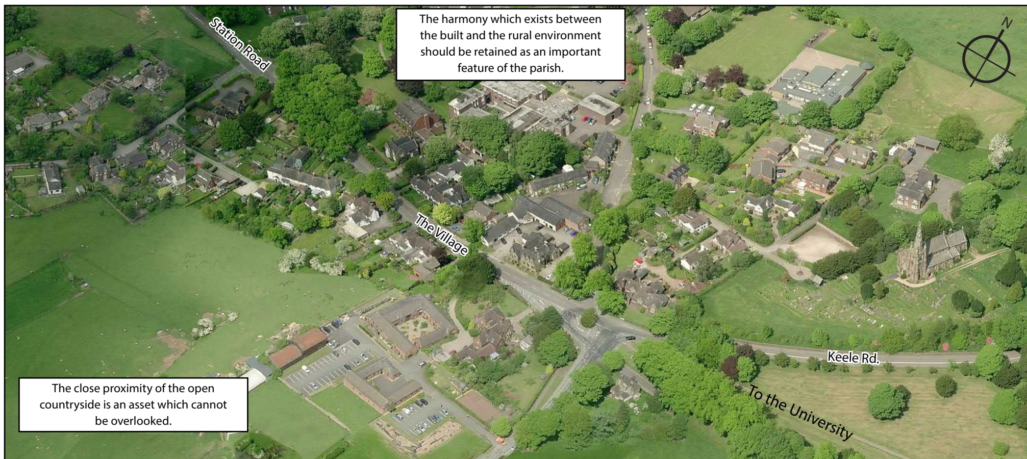
Figure 22: Aerial of the Village. The rural, landscaped nature and informal development style should be preserved.
