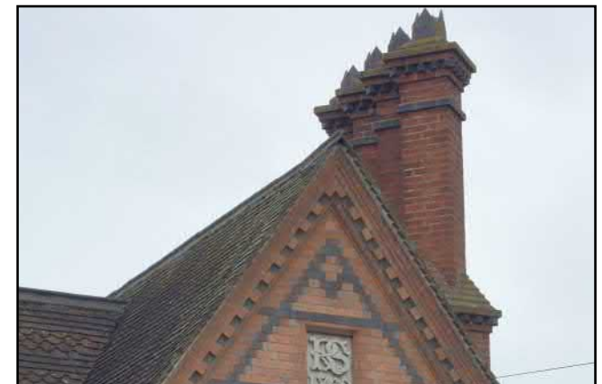
Figure 19: A highly textured and attractive building style.
