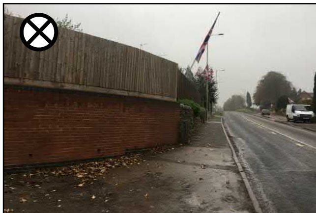
Figure 48: Panel fencing is out of scale and unattractive
