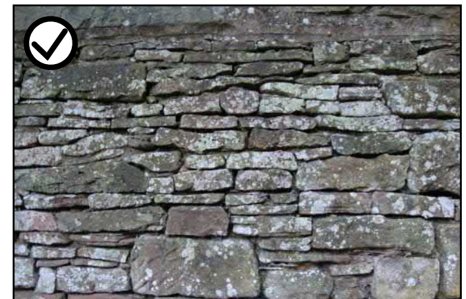
Figure 49: Traditional stone walls
