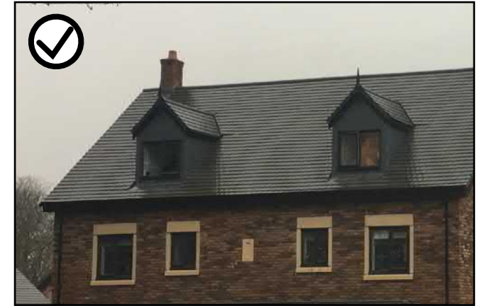
Figure 29: Appropriately sized dormers at The Hawthornes
