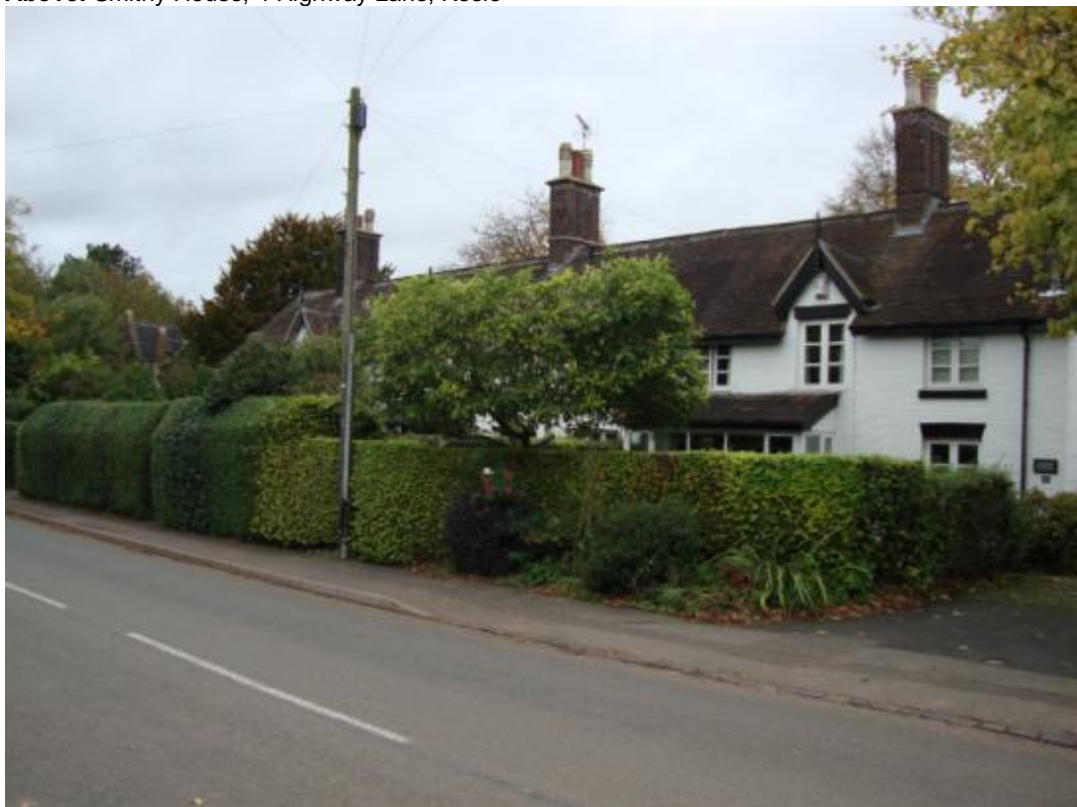
Above: The Cottages, 3-9 The Village, Keele. Well-clipped hedges are a strong characteristic of the village. This also reflects the pattern of development, complementing the alignment to the road that many properties have with the historic core.
