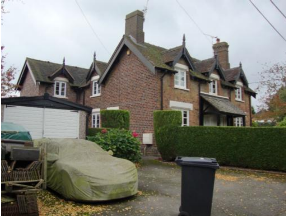
G: Building on the corner of Highway Lane and Pump Bank View 1
